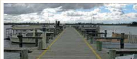
Berthing at a jetty
